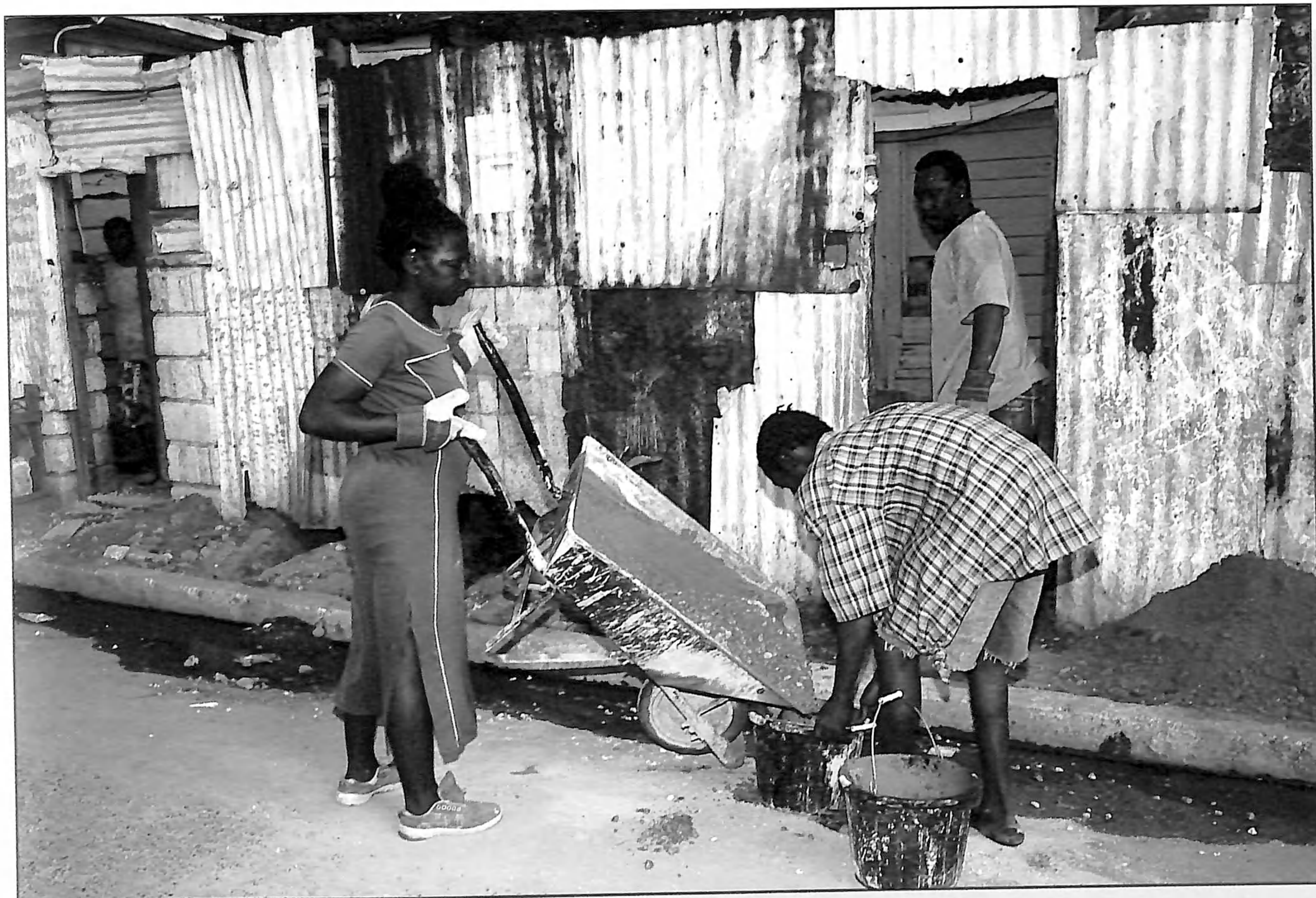
Construction project in the Caribbean.
